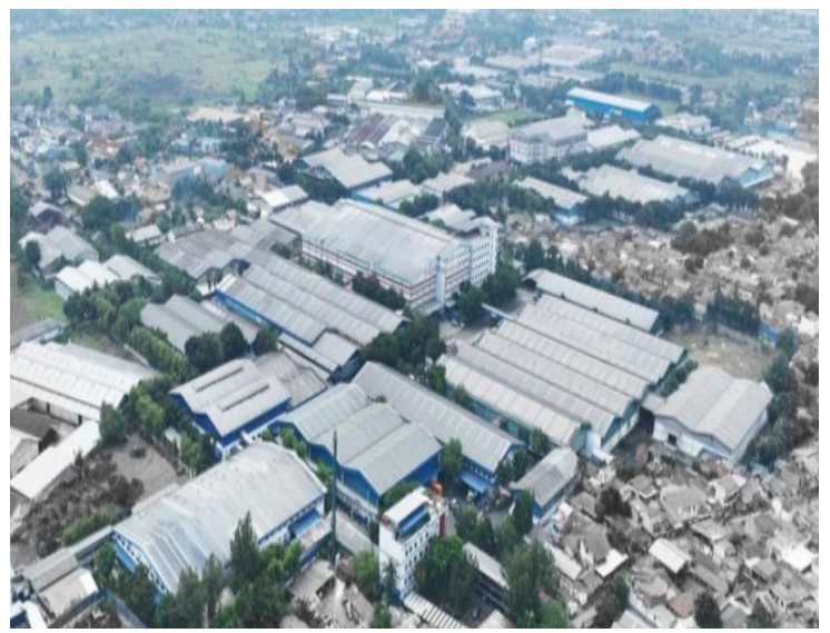
Figure 25: SMSM's production facility in Tangerang
